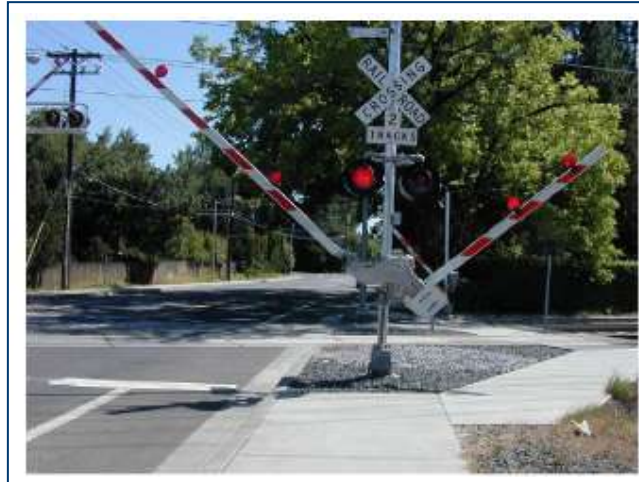
Figure 12 Example of a Pedestrian Crossing Gate
