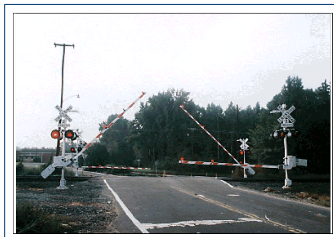
Figure 13 Example of a Four-quadrant Gate Crossing
